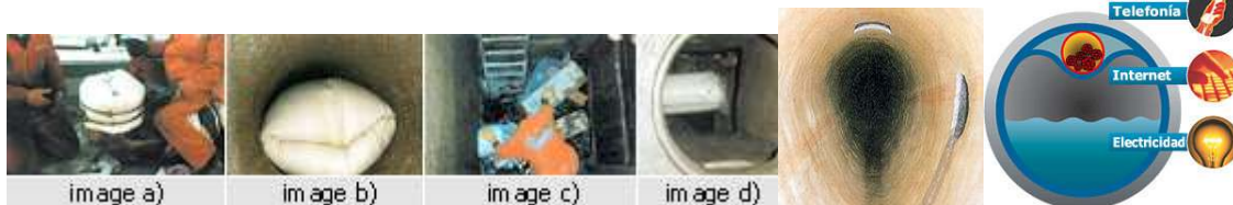
Positioning in-situ total sleeve including superior space for other conductions
