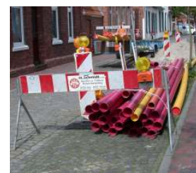
works in the street
